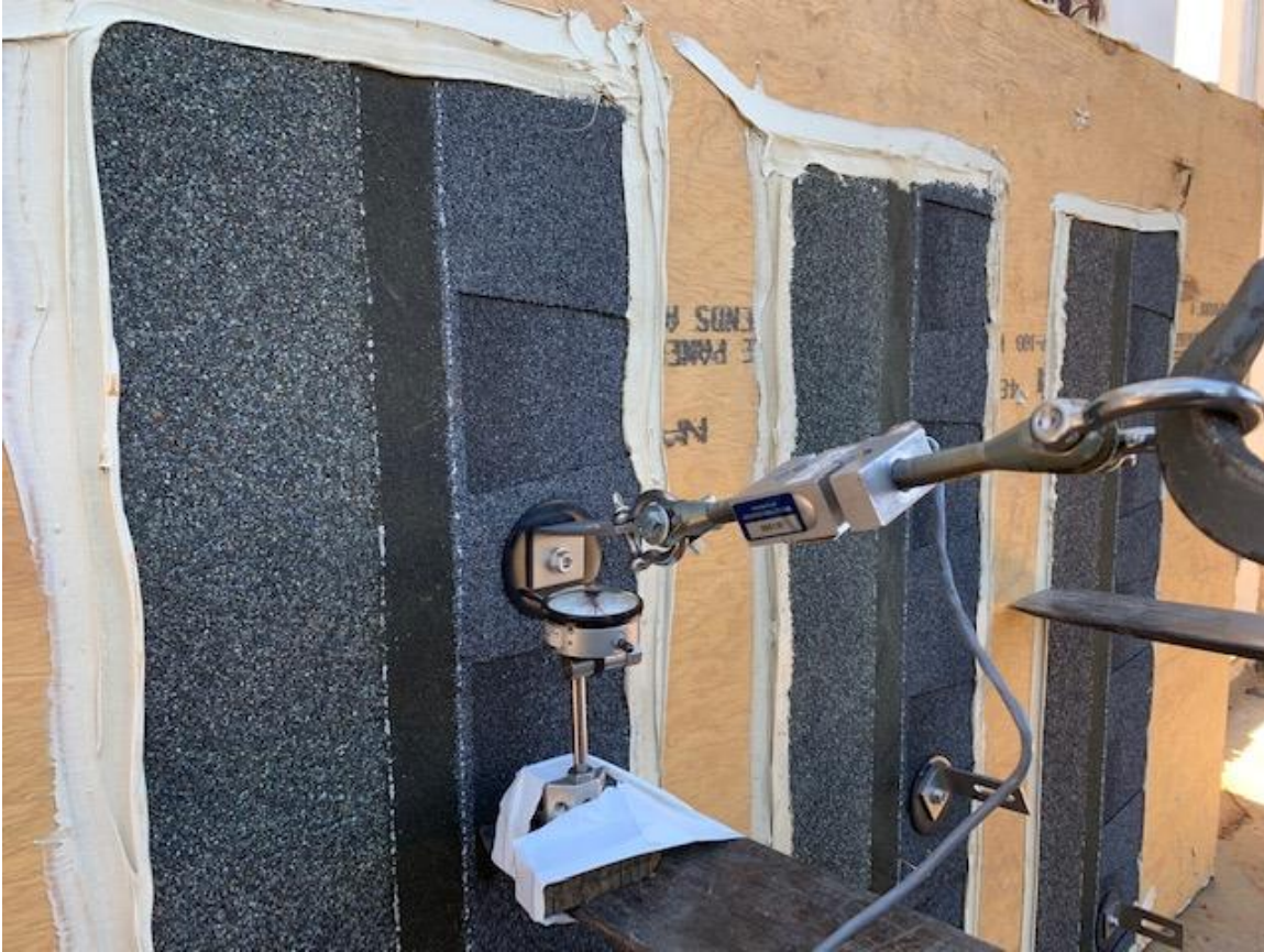
Photo No. 1 Pullout Test
